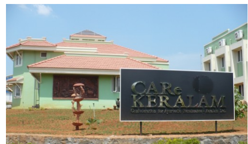
CARE Keralam complex, Thrissur
