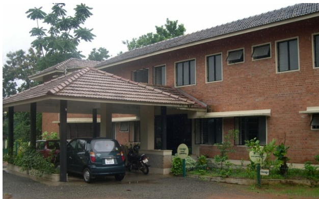
100-bedded district government hospital, Thodupuzha
