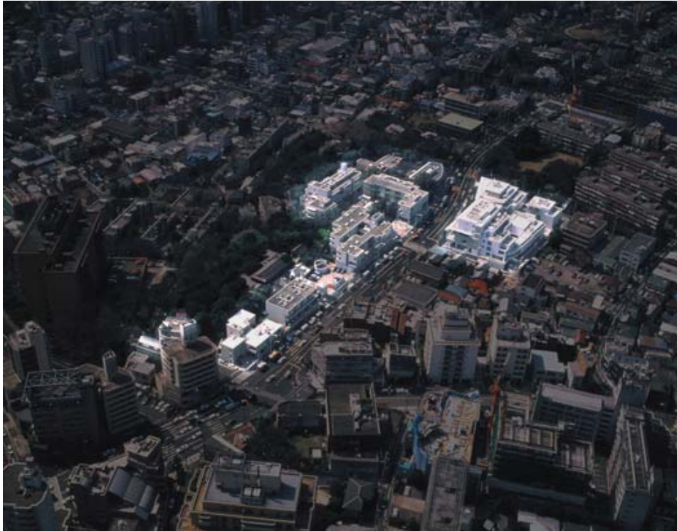
Figure 10. Fumihiko Maki, Hillside Terraces (1967-98)
