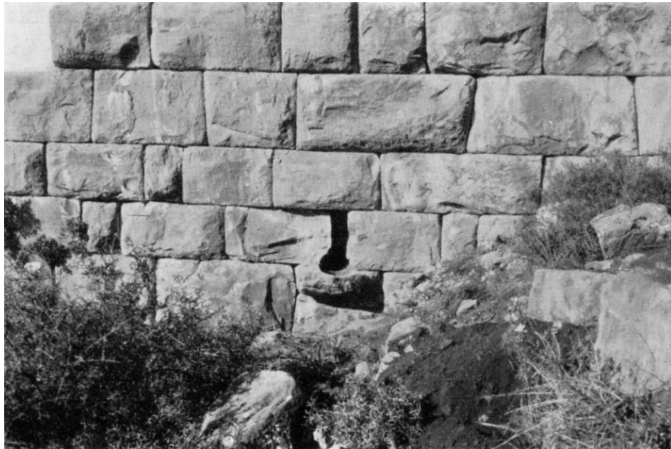
Fig. 27 Entrance of the water pipe through the city wall at Priene (Schede, Kleiner, and Kleiss, p. 22, fig. 22)
