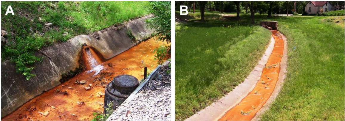
Figure 1-1. (A) In Belleville, IL, emerging groundwater is collected by French drains and discharged from a 6 inch pipe into a storm-water ditch where the precipitation of orange-colored iron oxide minerals is apparent. (B) The water flows and deposits minerals for about 0.5 miles through residential areas before entering a nearby creek.
