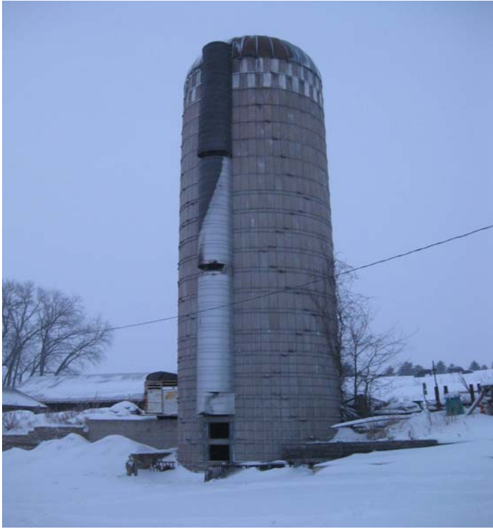
Figure 3.1 A typical silo on a farm
