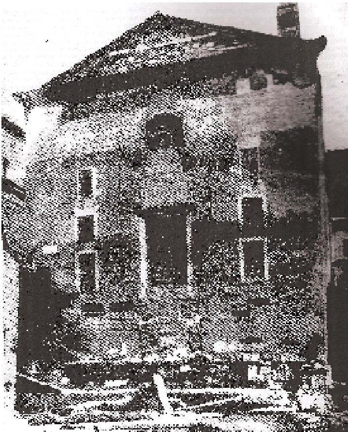
Front façade of the Diocletianic rebuilding of the Curia Iulia after Boni's restorations
