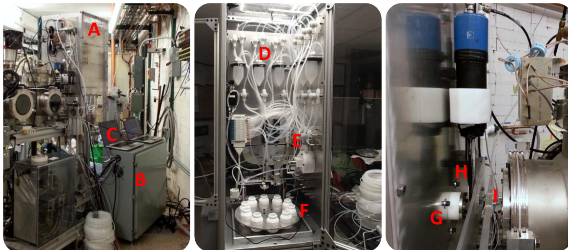
Figure 3-3. Photographs of the water cell collection end-station. (Left) Installation in the vault where the beam enters from the left, A is the side of the isolation box that holds the target cell and associated plumbing (see Fig. 3-2). B houses the electronic controls and C is a laptop that controls the system. (Center) Side view of the target end-station that shows D : the water reservoir system, E : the PTFE target cell and F : the rotating collection bottle system, (Right) Close up of the end of the beam line and G : water cell window, H : a removable scintillator in front of the target assembly, I : beam collimator.
