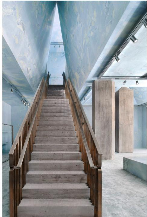
Architect: Valerio Olgiati **Owner:** Celine Year of completion: 2018 Climate: Tropical monsoon climate Application: Exterior and interior Properties of material: A marble shell is laid over an existing two-storey structure. The facades, floors, walls, ceilings are entirely made of marble. The blue-green Pinta Verde from Brazil is exceptional and creates a wonderful atmosphere for Céline.
