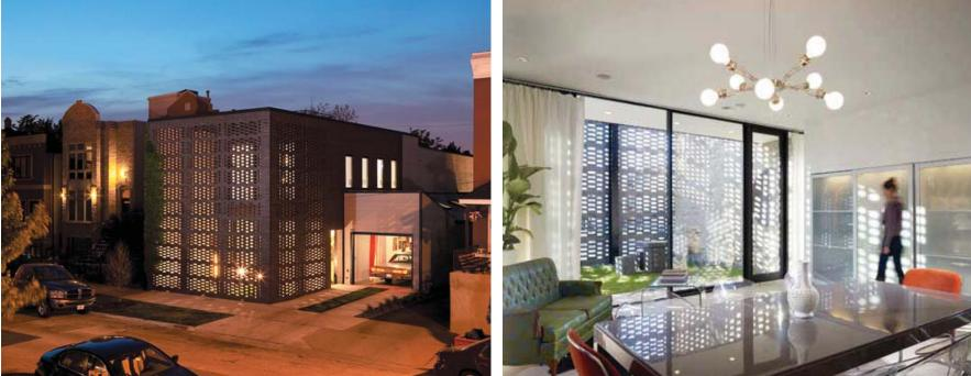
Architect: Studio Gang Architects Owner: Private Owner Year of completion: 2008 Climate: Humid Continental Material of interest: Brick Masonry Application: Exterior Screen Properties of material: Reused brick from the pre-
