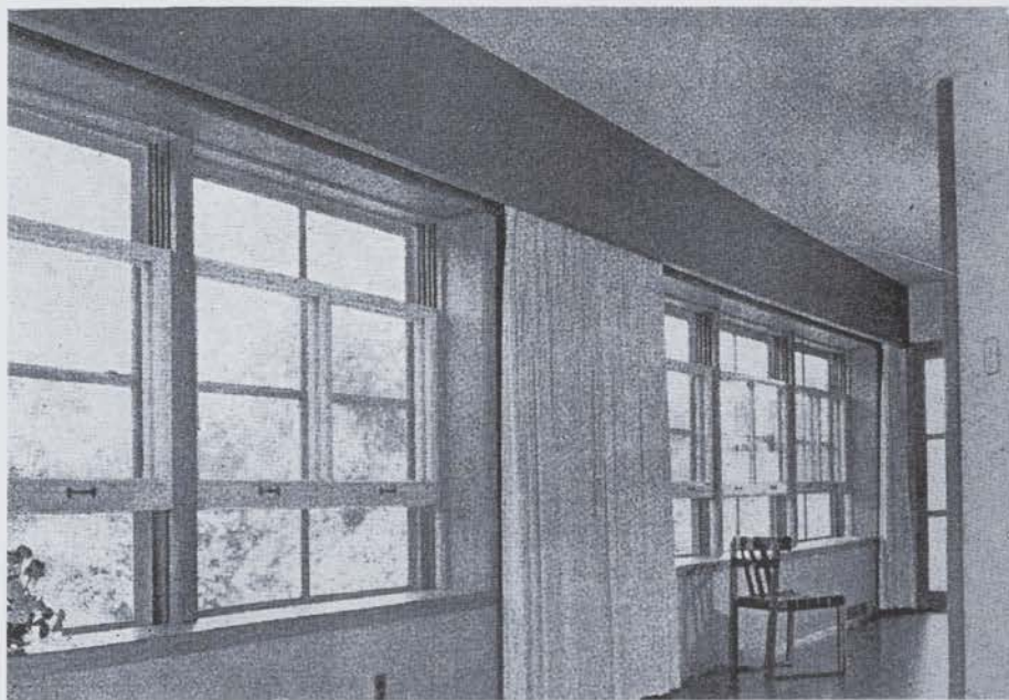
Fig. 44. Harris Armstrong House, window wall (north wall) joining living and dining room, showing ledge for informal seating.
