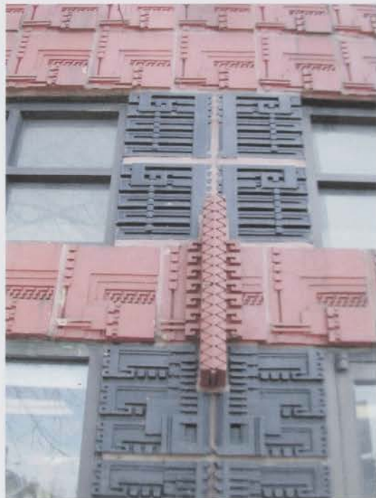
Fig. 19. DeBaliviere Building, exterior terracotta block detail.
