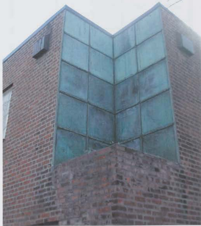
Fig. 34. Grant Medical Clinic, alley (north & west elevations), detail.
