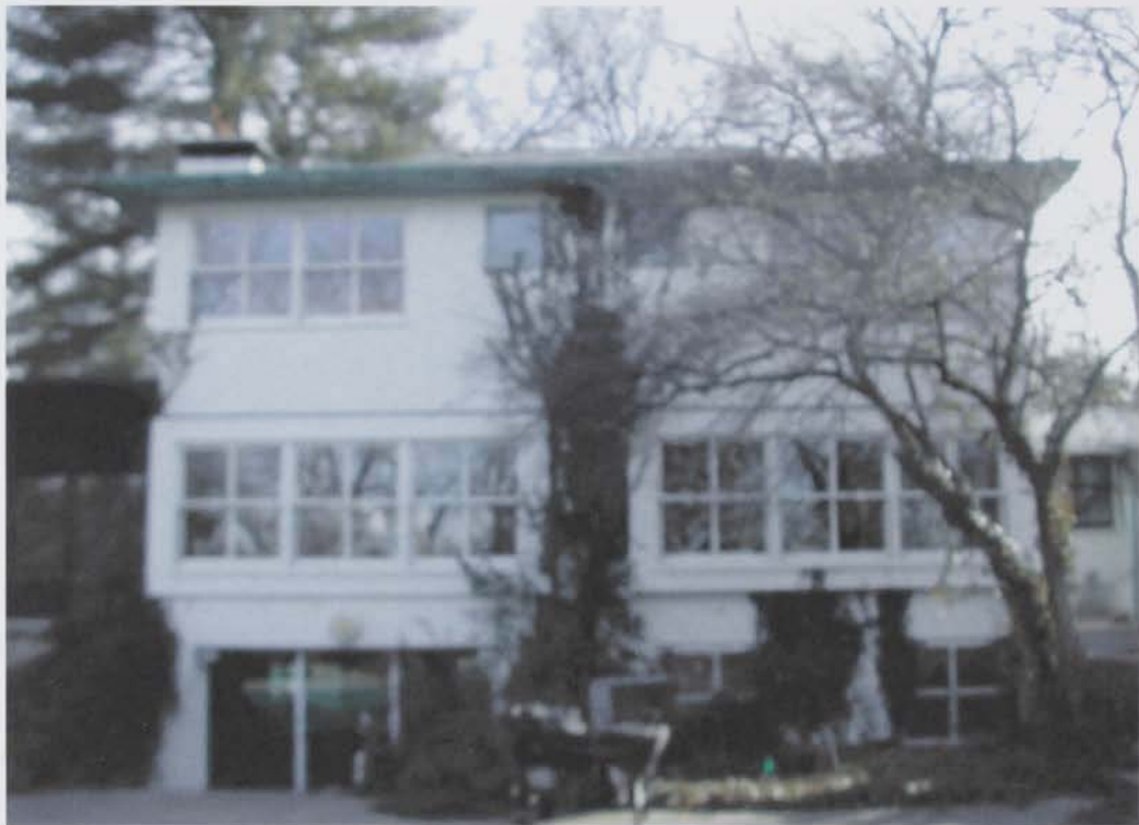
Fig. 43. Harris Armstrong House, back (north) elevation.
