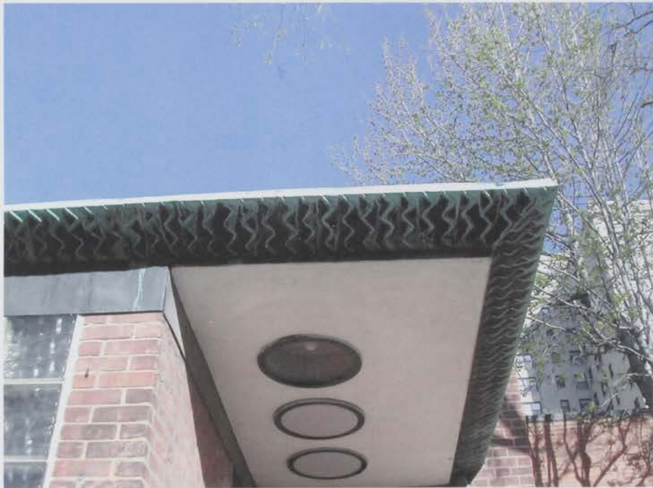
Fig. 40. Grant Medical Clinic, copper gutter detail.
