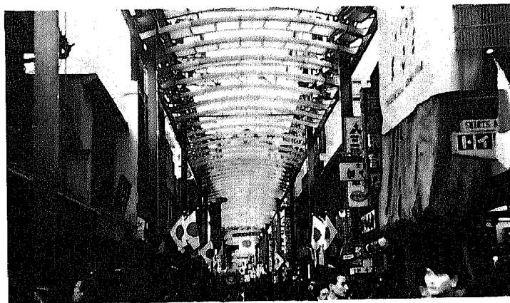
Fig. 15, (above), Shopping District in Shinsaibashi, Osaka: A roof unifier which is becoming more and more common in Japan. Each shop pays a portion of the cost of the structure. The roof simplifies and unifies streets which are otherwise chaotic. This elaborate example of mediation moves as the weather demands.
