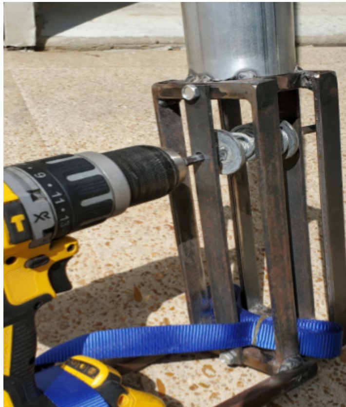
Figure 31: Close up of bottom box and steel tubing
