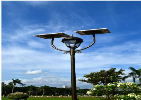
Fig4.2 Solar cells street lamp
