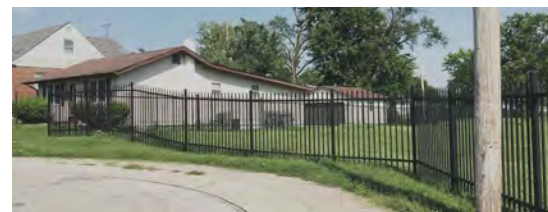
Fig 2.6. Detention basin fence
