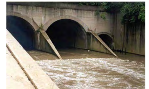
Fig 2.9. Vaulted brick sewer arch
