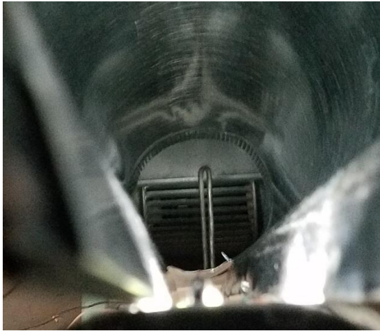
Figure 18: The setup for testing the water heater element viewed through the duct nozzle opening.
