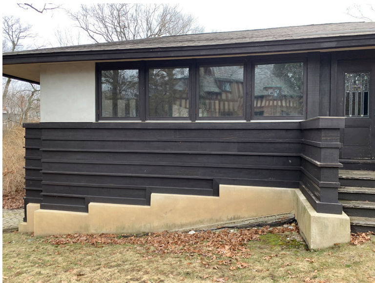
Figure 5.3. Glasner House. Exterior view, enclosed porch and garage from the South. The slope of the ground is echoed in the stepping of the concrete base. Photograph by author.
