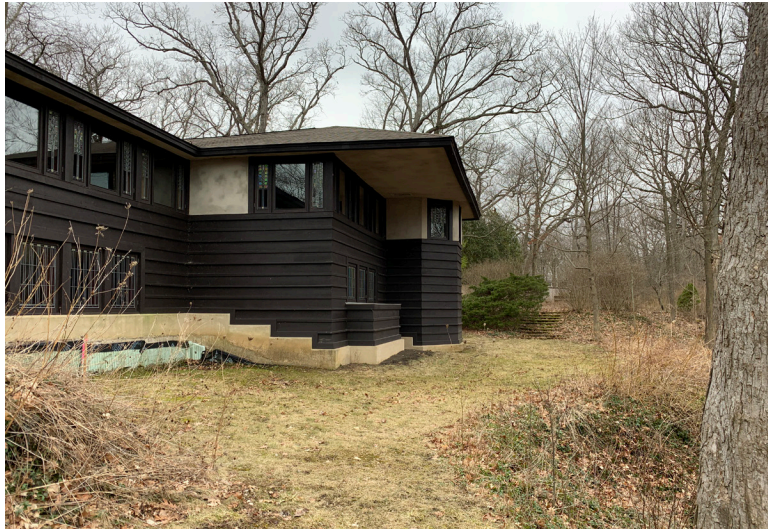
Figure 5.2. Glasner House. Exterior view from “table ground,” looking southwest. Modifications to the slope of the terrain are evident at the concrete base. Photograph by author.
