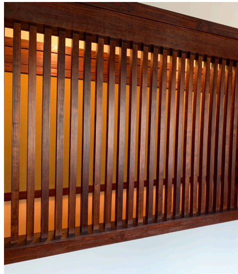
Figure 2.18. Glasner House. Detail of wood screen between kitchen and basement stair. Photograph by author.
