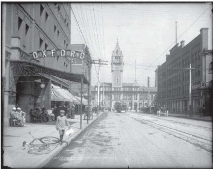
Figure 5.3 - Block 14 to the left, Block E to the right
