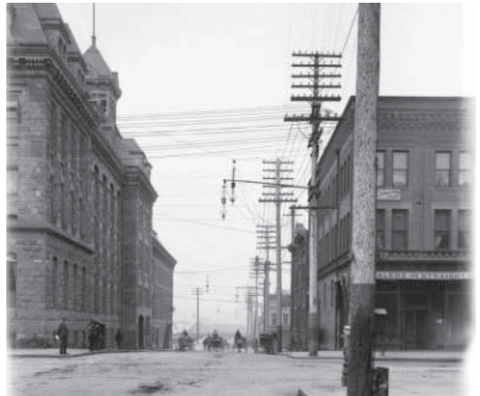
Figure 5.5 - Blocks 44 and 45 looking north on 14th Street
