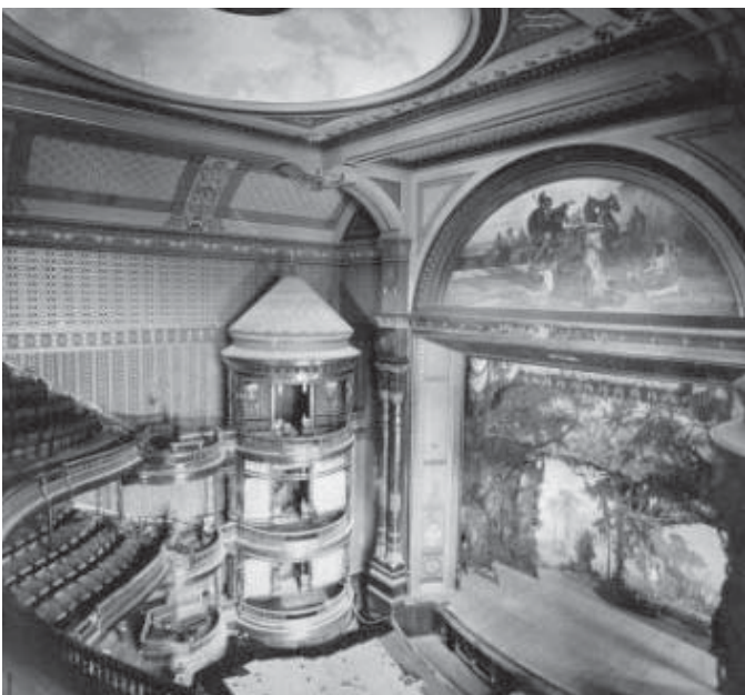
Figure 7.3 - Tabor auditorium interior
