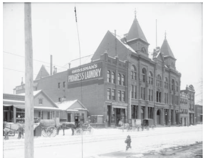
Figure 5.13 - Block 92, northeast corner of 22nd and Arapahoe Streets
