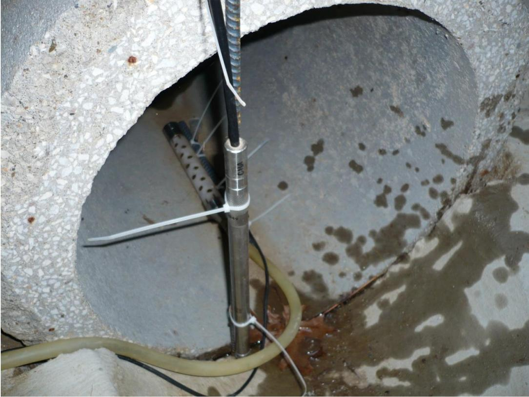
Figure 2.3. Typical in situ water level sensor field installation in a storm sewer to measure runoff water level.
